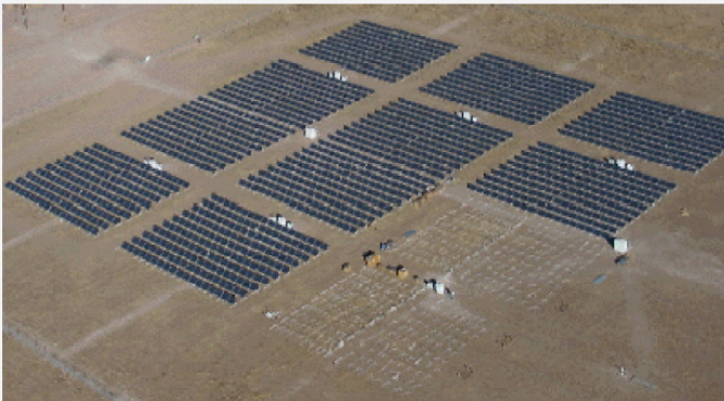
Photovoltaic Power Plant, Tucson Electric Power Co., Arizona Nominal Power (August 2002): 2.4 MW Photovoltaics: Multi-crystalline Silicon (ASE), CdTe (BP-Solar), amorphous Silicon
